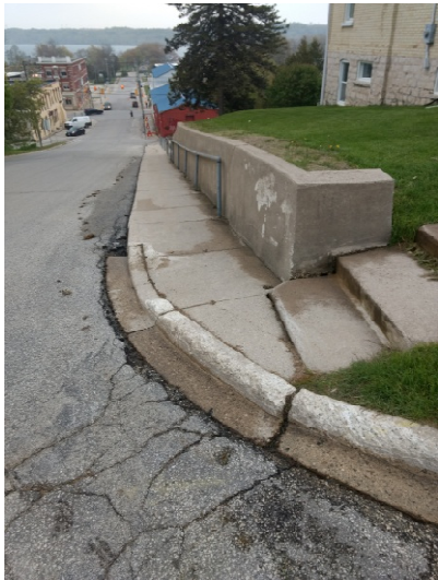
Trip 88 - stair landing
