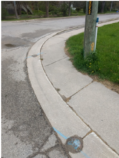
Trip 20 - Curb at Intersection Example
