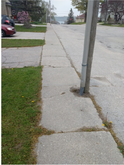
Trip 82 - After cleaning grass and dirt potentially example
