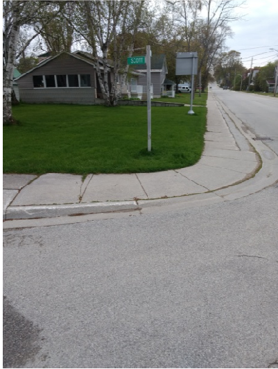
Trip 26 - Curb at Intersection Example
