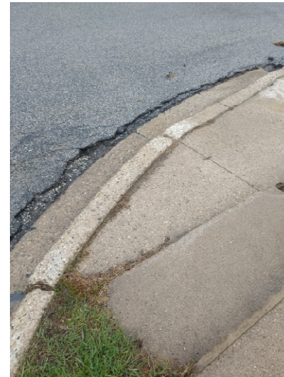
Trip 111 - At Curb Entry
