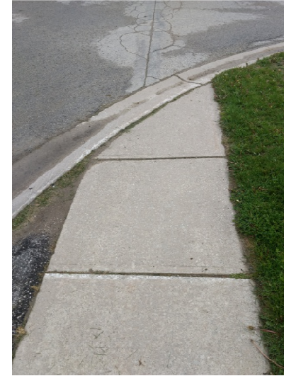
Trip 19 - Curb at Intersection Example
